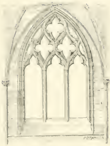
FLOWING TRACERY, WELLS CATHEDRAL.
